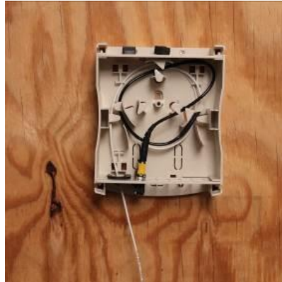
MTP terminated InvisiLight Multifiber Cord plugged into Slimbox 12 fiber MDU terminal Options for SC and LC are also available.
