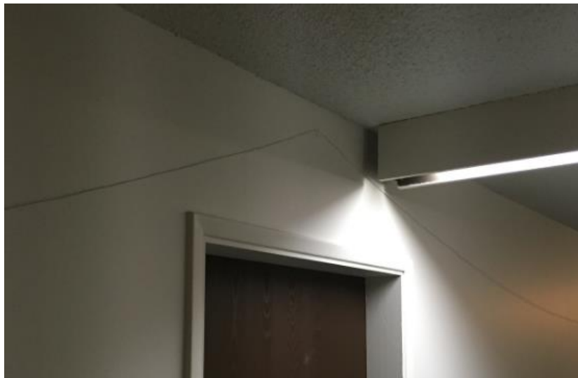
InvisiLight Multifiber Cord supported by a clip above a doorway before it is adhered to the wall
