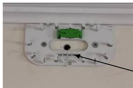
Point of Entry module pre-installed on a wall
